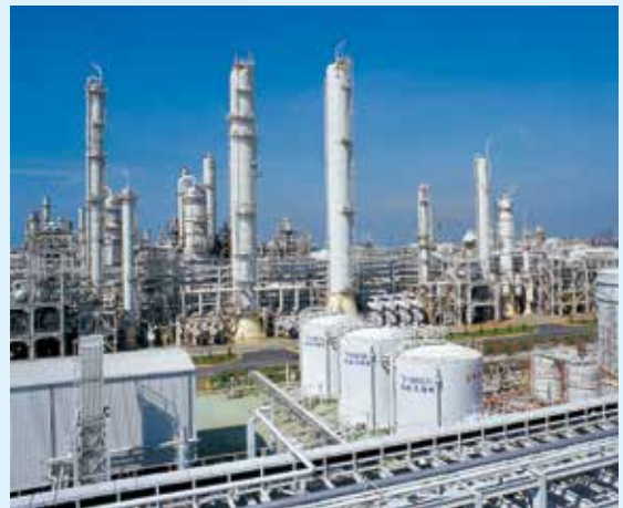
工廠排水配管 Petrochemical plant
