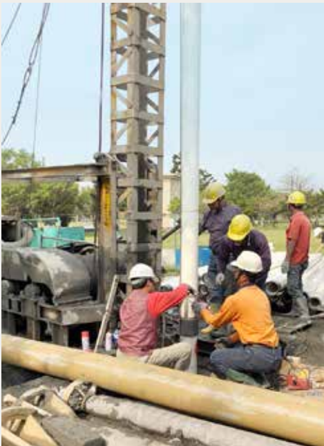
鑿井工程 Well drilling engineering
